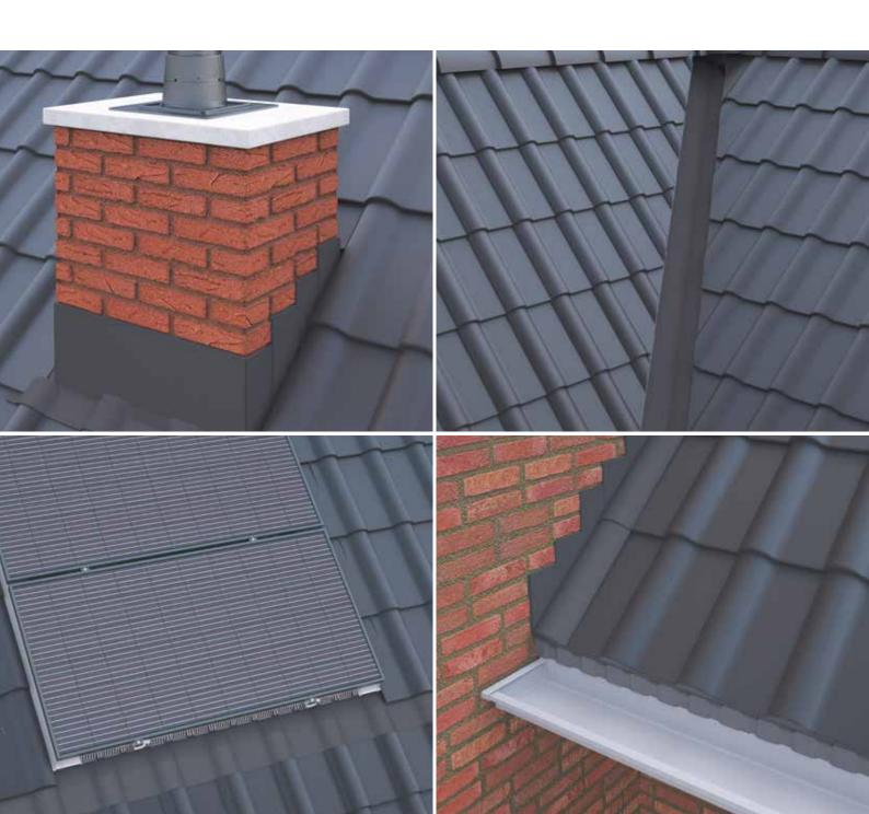
Ubbink's non-lead waterproof flashing range provides practical, easy-to-install solutions for applications where lead is traditionally used, such as changes of direction and materials. With no lead, they have no scrap value and are therefore an ideal way to combat the perennial problem of lead theft from roofs.
