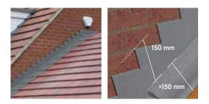
Alternatively, single lap tiles can be weatherproofed at abutments by using a cover flashing and a separate stepped flashing (figure 07). As in double lapped tiles, the cover flashing should run 75mm up the wall and the stepped flashing should be 150mm
